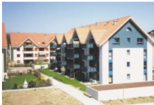
Baustelle in 3270 Aarberg
